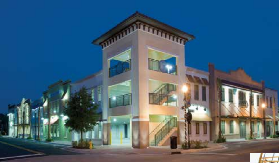
Decorative touches, ranging from brick and tile to awnings, cornices, and colorful paint, create the look of retail storefronts for a new precast concrete parking structure in downtown Winter Haven, Fla. Panels were overlapped to create a varying rhythm to the façade, and a variety of lighting fixtures minimize light overflow and mimic retail appearances. Photo courtesy of Mike Potthast, Potthast Studios
