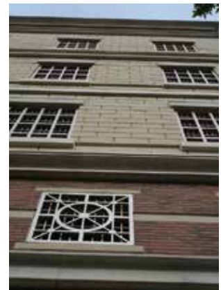
A traditional tripartite design with faux windows and elaborate details, including embedded thin brick in the architectural precast concrete panels, help the façade of the Central West Garage in Lancaster, Pa. fit in with its neighbors. The all-precast concrete structural system was connected on each level with an existing adjacent parking structure.
