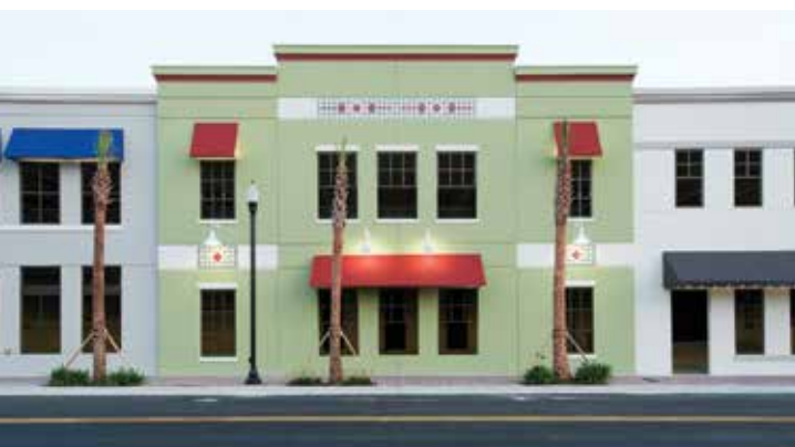
Photos courtesy of Everett Whitehead & Son, Inc.
