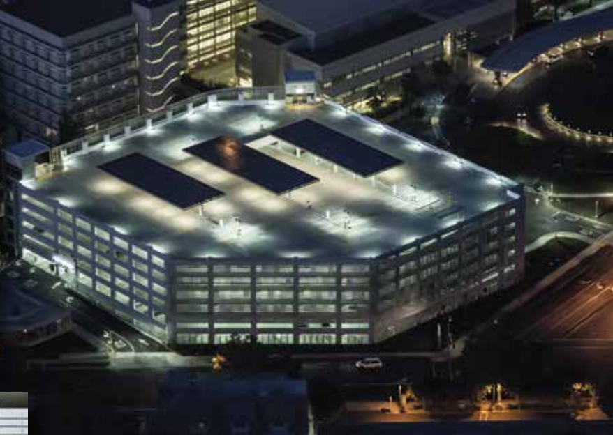
The high-profile parking structure at the UC Davis Medical Center in Sacramento features aluminum louvers and other metal decorations attached to the precast concrete spandrel panels. Each set of louvers is angled slightly differently, to cast different shadows through the day and imply movement.
